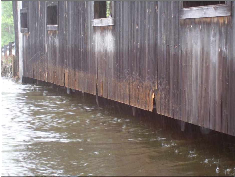
Joppa Covered Bridge over Warner River
