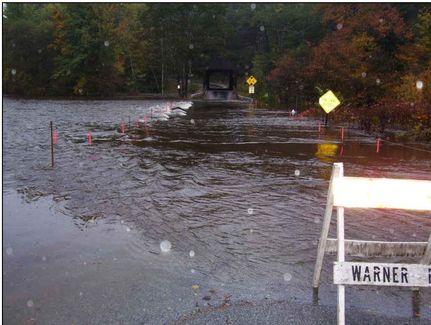
Warner River Overflow onto West Joppa Road to Covered Bridge
