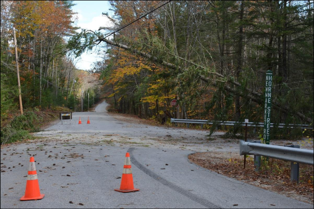
Horne Street and Newmarket Road Intersection – Tree Down on Wire, October 2017
