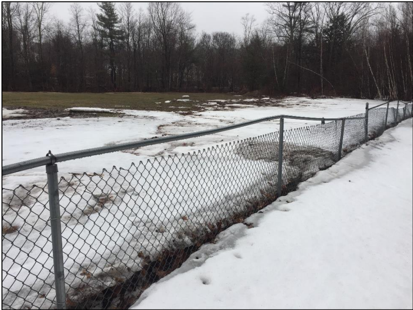
Riverside Park Baseball and Softball Fields Fencing, January 2018
