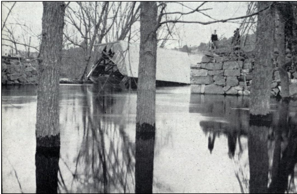
Webster Bridge in Davisville
