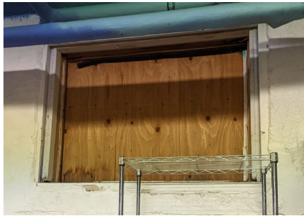
Photo 2. Uninsulated, leaky loading window
