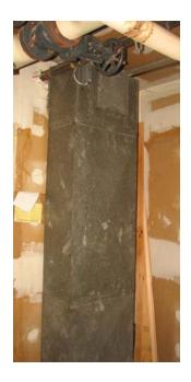
3.) The combustion air assembly serving the boiler does not appear to meet code.
