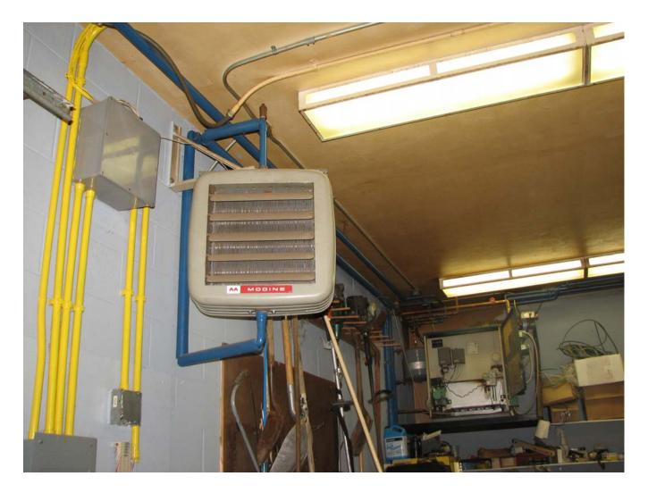
**Distribution –** modine space heater (above) and FHW baseboards in office and labs. **Boiler** Valiant Propane - Atmospheric 134K Input Net IBR 116,500 Approx 86% combustion efficiency
