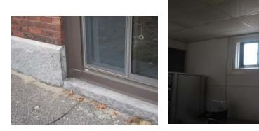
The above pattern suggests water leakage – probably in the past – and perhaps before exterior patching below the window. Gutting this area of wall to make sure all has effectively dried is advised for building durability and health benefits. Woodwork may make retrofitting this stairwell area cost prohibitive, however air sealing the window opening and adding an interior, air tight, storm, is recommended.
