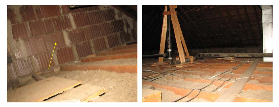
Attics are a great place to see construction materials used the building but which may be covered. The ceramic tiles above can also be seen in a wall cavity in the basement and behind the stairs in the large stairwell.
