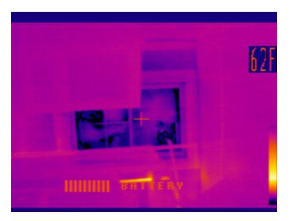
Windows can leak air wherever the sash or unit ends and the rough opening or trim begins. All of it can be sealed.
