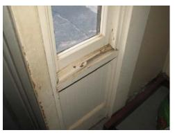
Effective air sealing requires removing all trim and sealing the rough opening around the window unit, as well as the sashes themselves.
