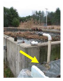
This line has been insulated but also uses a heat tape to prevent freezing – especially where it enters the reed beds where it is most unprotected.
