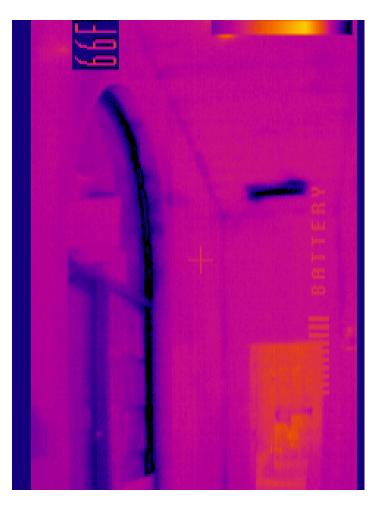
Window rough opening sealing is called for. Access to above top plates from attic above.
